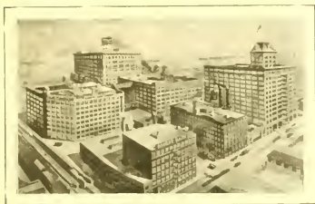
A group of factories built of concrete, in Brooklyn. Paper goods are manufactured here.
